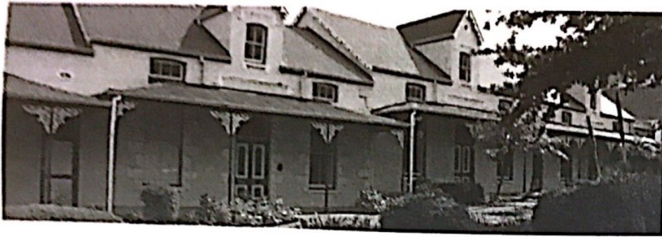
18-24 Crozier Road, home of the Law Clinic since December 2017. PHOTO: SU Corporate Communication.
